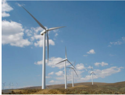
FIGURE 6.57 Horizontal axis wind turbines.
