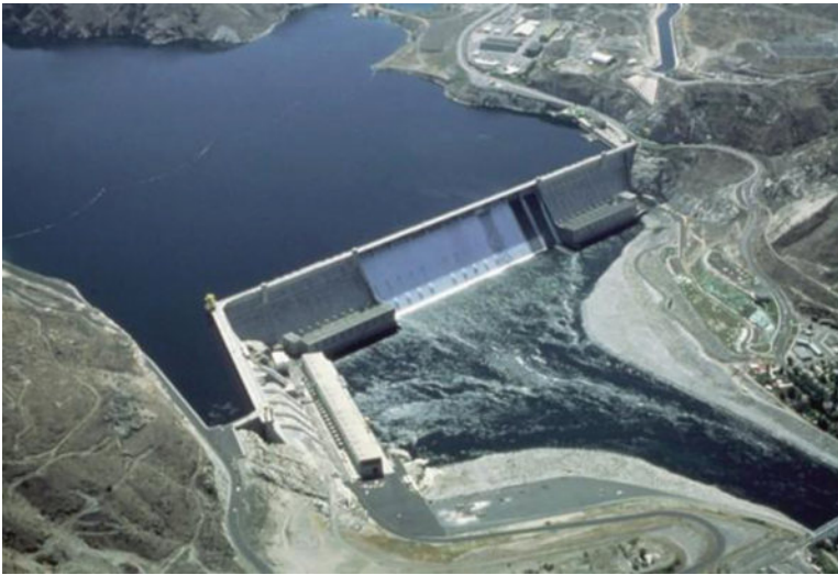
FIGURE 4.1 The Grand Coulee dam and Franklin D. Roosevelt lake. (Image courtesy of U.S. Army Corps of Engineers, Louisville, KY.)
