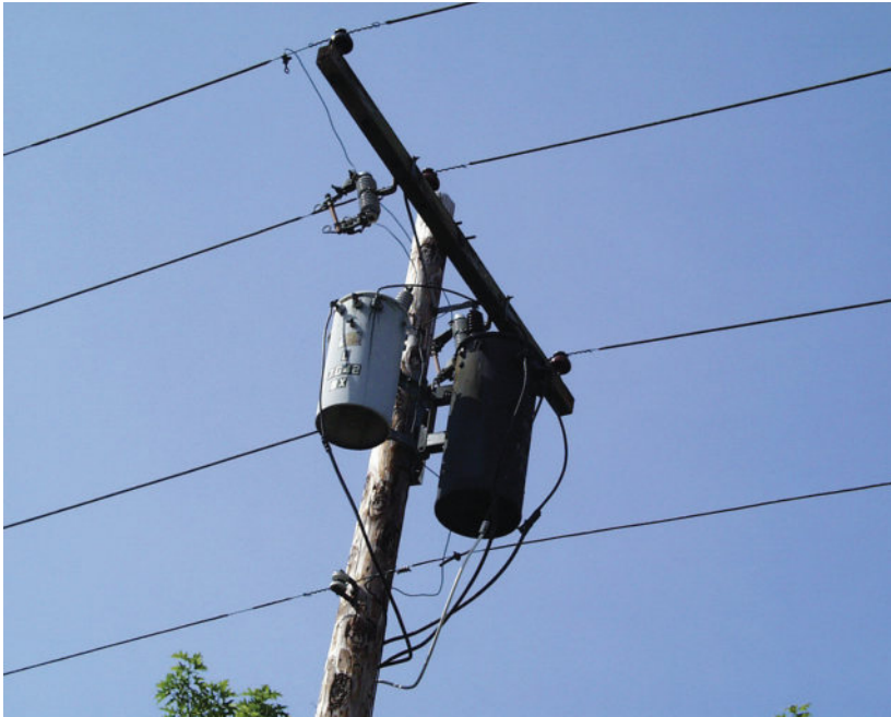
FIGURE 8.8 Single circuit distribution line.
