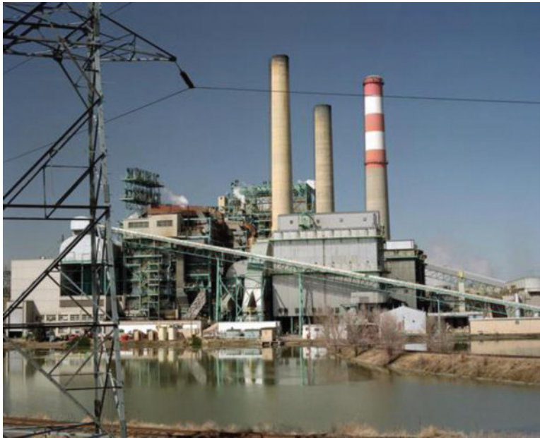
FIGURE 4.19 Weston coal-fired power plant. (Image courtesy of the U.S. Department of Energy, Washington, DC.)
