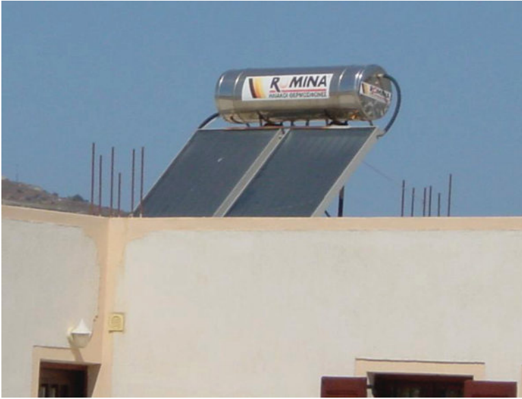
FIGURE 6.5 Passive thermosiphon hot water solar system.
