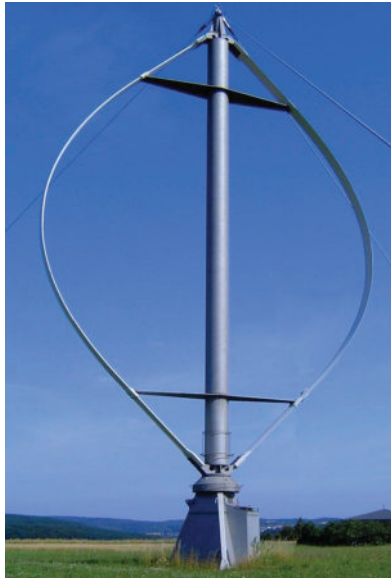
FIGURE 6.59 Vertical axis wind turbine. (Courtesy of US National Renewable Energy Lab.)
