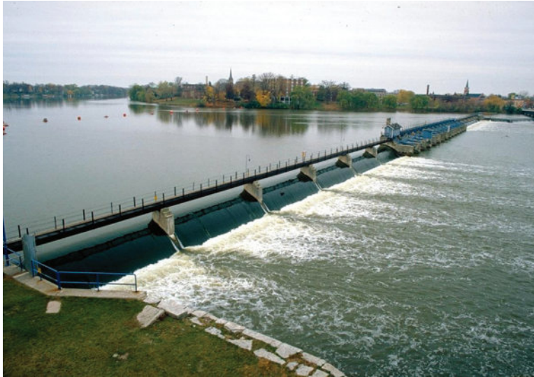
FIGURE 4.2 Fox River diversion hydroelectric power plant, Wisconsin. (Image courtesy of U.S. Army Corps of Engineers, Louisville, KY.)
