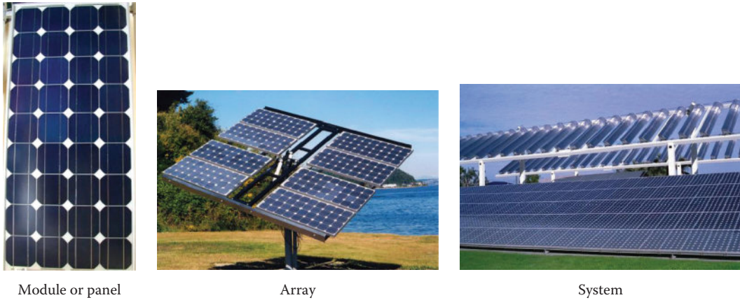
FIGURE 6.25 PV module, PV array, and PV system. (Images courtesy of the US Department of Energy, Washington, DC.)
