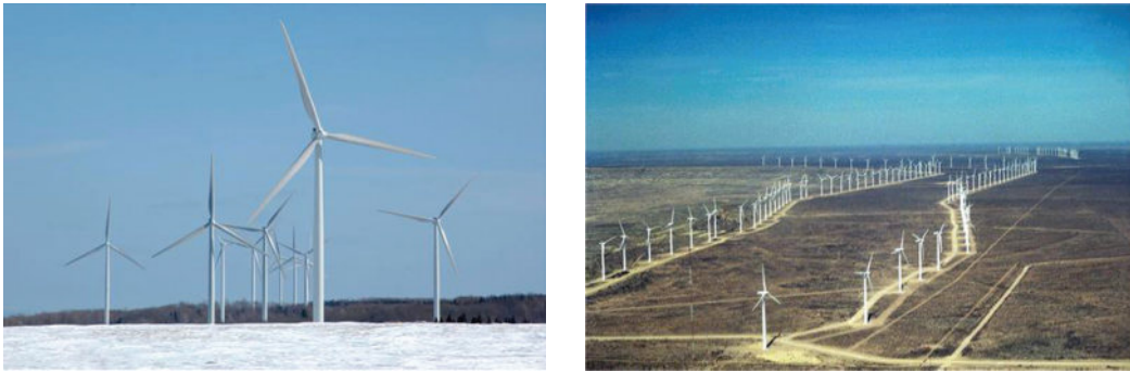
FIGURE 6.65 Wind farm located in California. (Images are courtesy of the U.S. Department of Energy, Washington, DC.)
